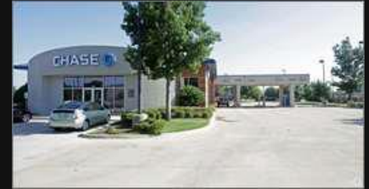
CHASE BANK Colleyville, TX Retail | 4.80% CAP | 4,225 SF
