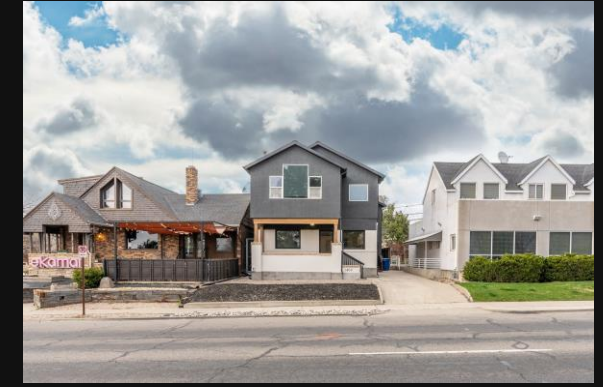
OFFICE Salt Lake City, UT Office | 9% CAP | 3,307 SF
